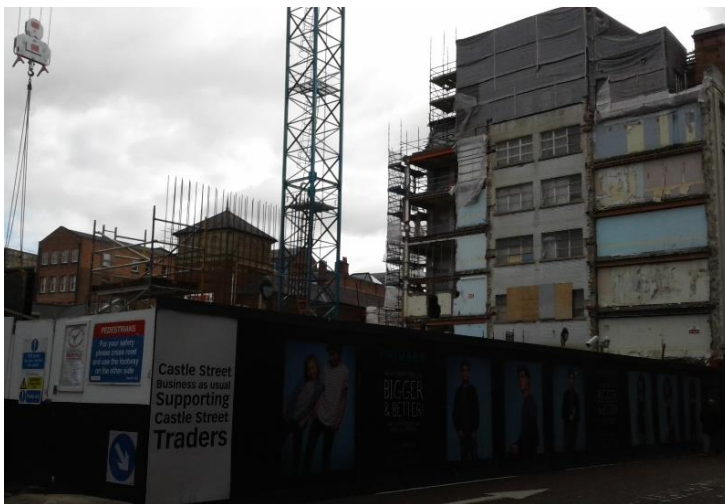
Commonwealth House, Castle Street (current works)
